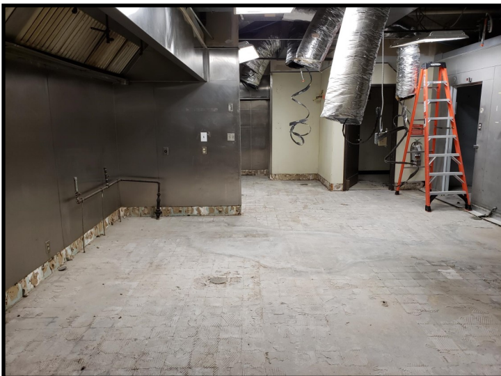
A view of the kitchen with all the tile flooring, ceiling, appliances, and equipment removed
