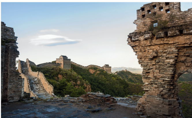
Sections of the Great Wall of China have been damaged due to age, earthquakes, and vandalism.
